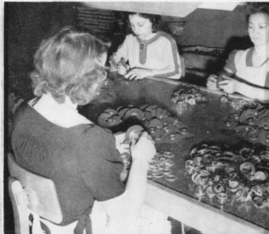
This young lady at Scovill's Schrader Division in Brooklyn, New York, checks an oxygen valve part under water. It just has to be perfect.
